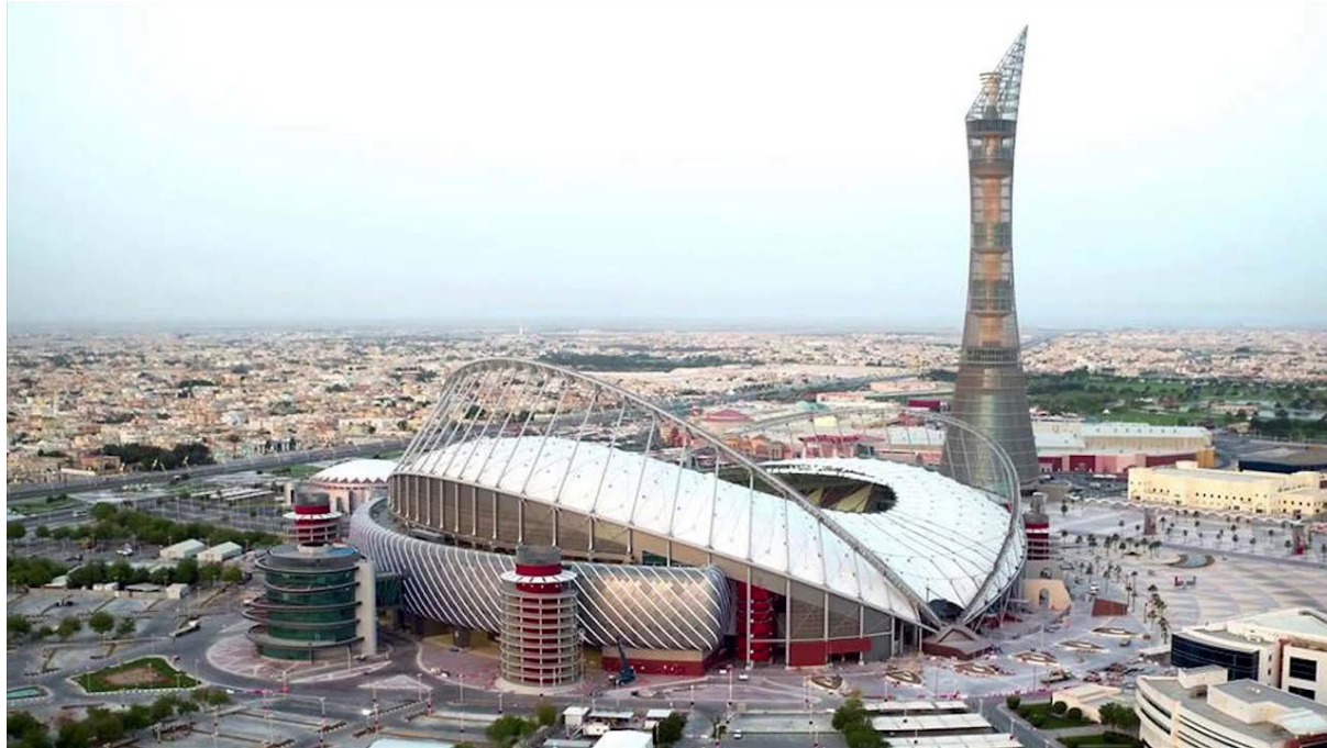
Exemplu: Khalifa International Stadium, Qatar. Sursa: timesofmalta.com
