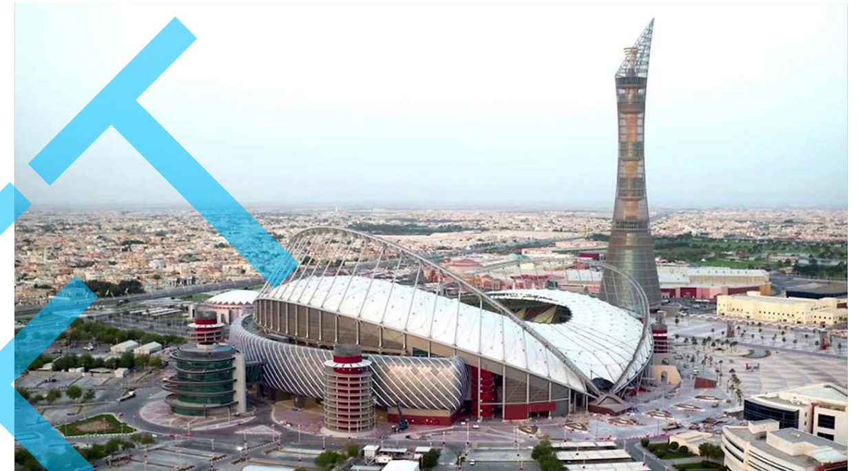
Exemplu: Khalifa International Stadium, Qatar. Sursa: timesofmalta.com
